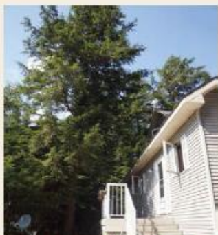
Figure A7-3. Conifer fuels overhanging a structure and deck (priority zone 1)
